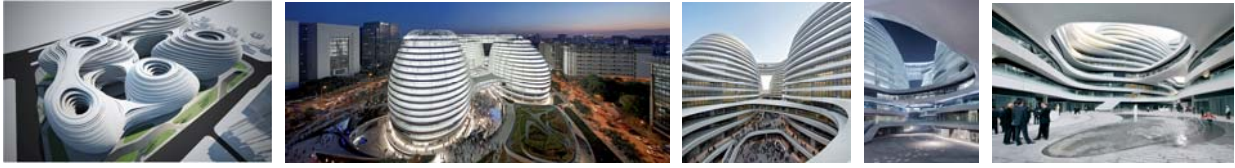
Figure 4. Multifunctional structure—Chaoyangmen Beijing SOHO III
