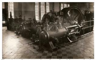
Fig. 1 Steam engine for electricity production (cogeneration) at Warsaw University of Technology [3].
