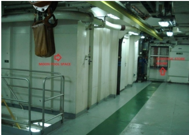
Fig. 6 Space for SOFC plant.
