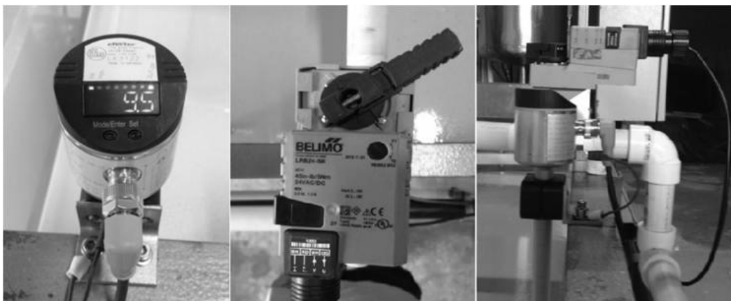
Fig. 5 Control elements (sensor and valve).
