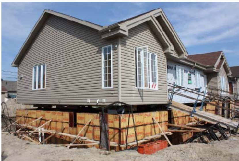
Fig. 2 Replacement of the concrete foundation walls.
