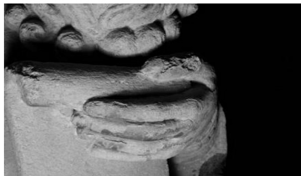
Fig. 1 Deterioration processes affecting the porch of the glory: arenization due to seritic alteration of the granite.
